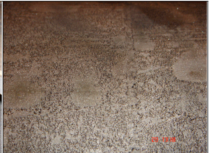
Close-up of steel after RPR induction
