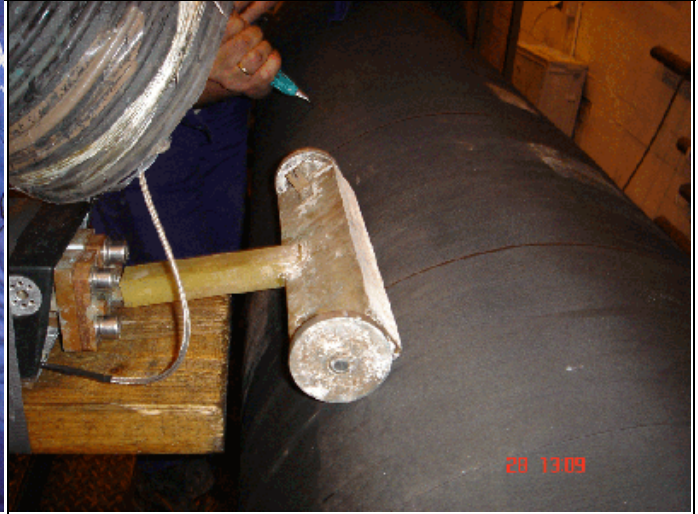
RPR induction unit in action
