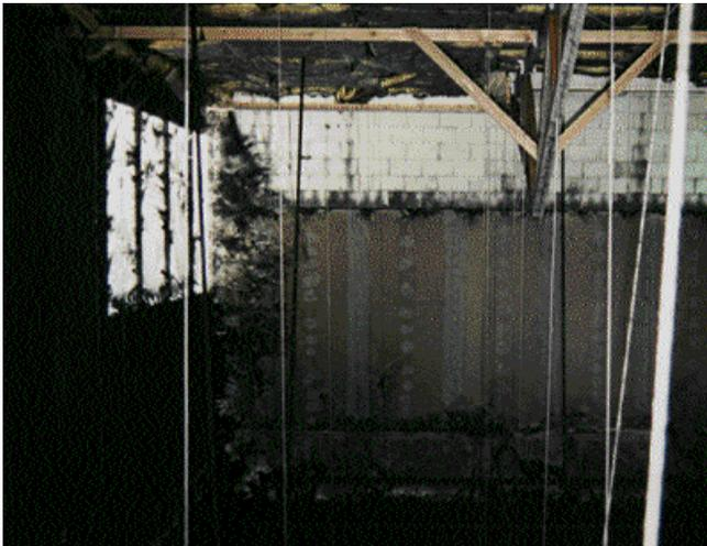
A production line fire at a Southeastern (US) Composite lamination factory left facility management and insurance adjusters with 32,000 ft<sup>2</sup> (2,973 m<sup>2</sup>) of black soot and odor to remove. The soot had to be removed from metal pan ceilings and trusses, concrete block and unpainted sheetrock walls - then from concrete flooring. Adjusters solicited bids to complete the project. A local area restoration contractor was awarded the job.
